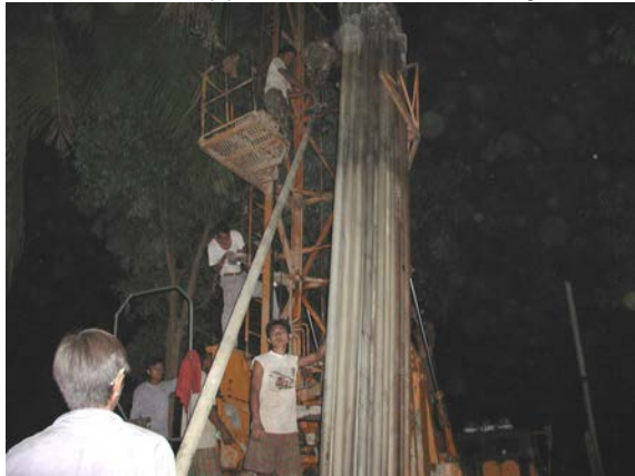
4"ø GI pipe installation at Twinma village
