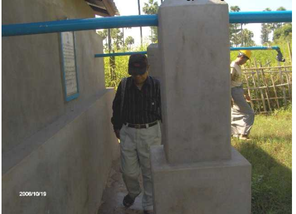
Auditor's site inspection at Htantawgyi village tubewell
