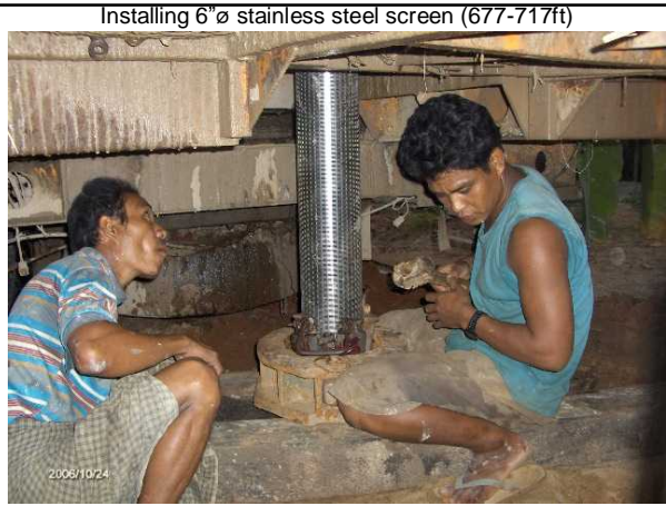
Installing 6" ø stainless steel screen (677-717ft)
