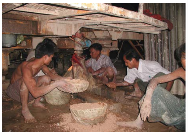
Gravel packing after pipe installation at Twinma village
