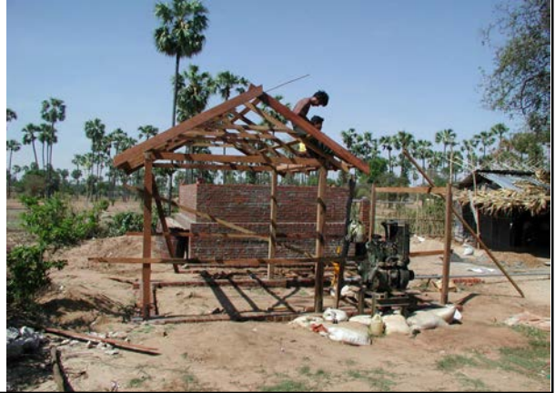
Carpenter work for engine house
