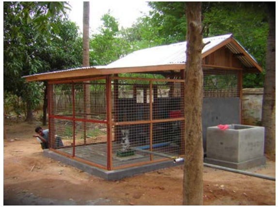
Completion of an engine house and a site tank
