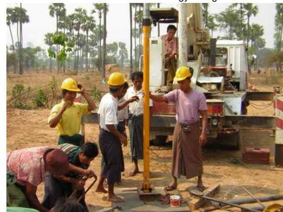
Mono element installation at Htantawgyi village tubewell
