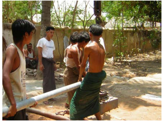
Villagers' participation at Twinma tubewell mono pump installation
