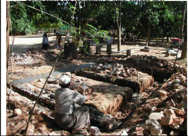
Constructing the foundation of water storage tank
