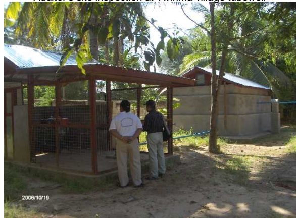
Auditor's site inspection at Twinma village tubewell
