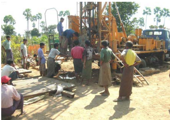
Tubewell drilling process at Htantawgyi village
