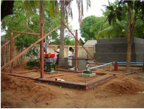
Carpenter work for engine house construction
