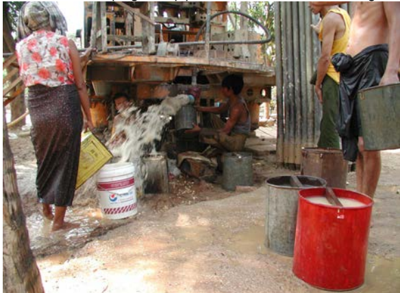
Tubewell developing after pipe installation at Twinma village
