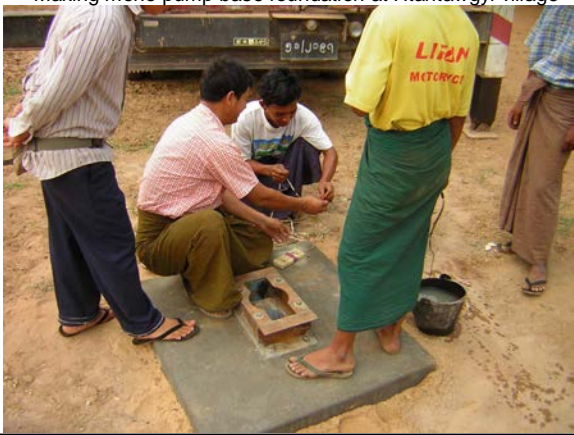
Making mono pump base foundation at Htantawgyi village
