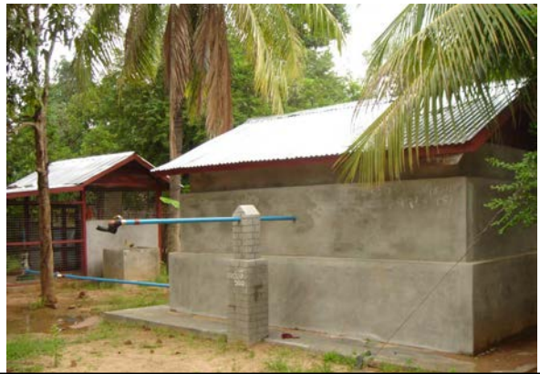
Completed water supply facilities at Twinma village
