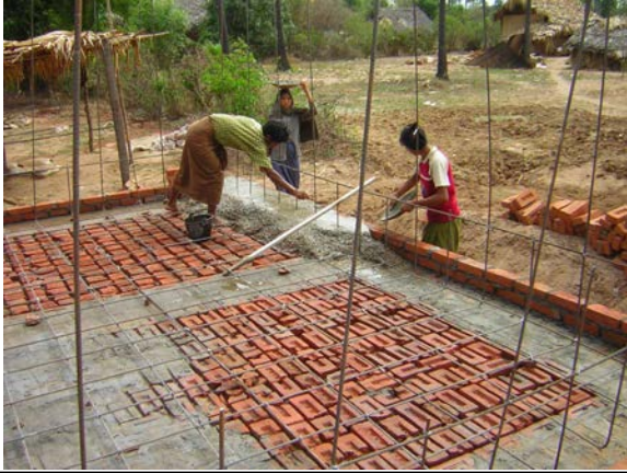
Constructing a 5,000 gals water storage tank
