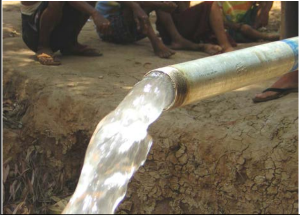
Pumping test after mono pump installation at Twinma village
