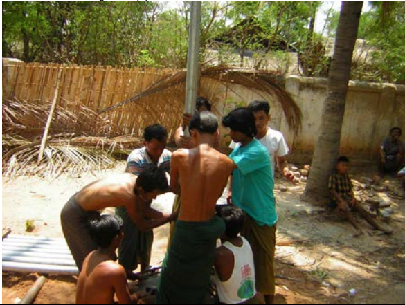
Installing mono pipes into the borehole of Twinma tubewell
