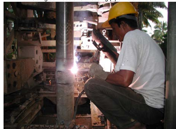
Welding services at 6" ø casing pipe installation
