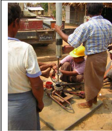
Installing mono riser pipes into the borehole of Htantawgyi village
