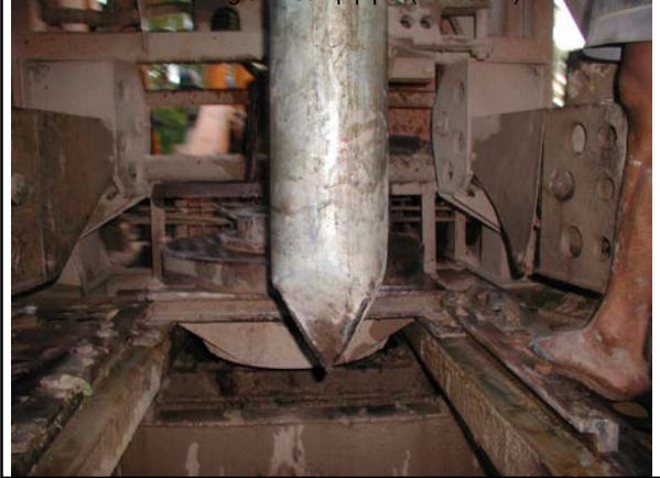
Installing 6" ø sump pipe (717-737ft)
