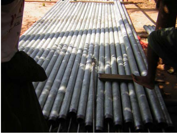
Mono pipes going to install at Twinma tubewell
