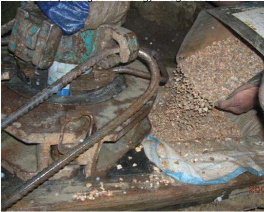
Gravel packing at Htantawgyi village tubewell
