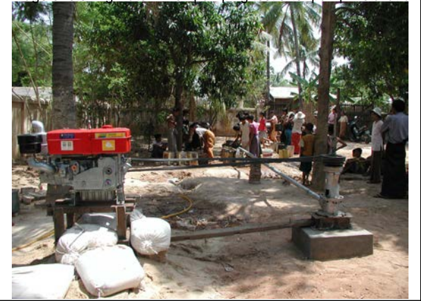
Villagers fetching water when pumping test after pump installation
