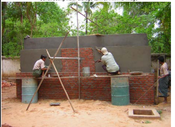
Constructing water storage tank at Twinma village
