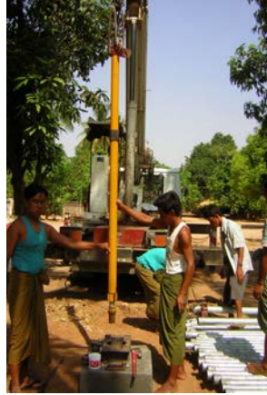
Installing mono element into the borehole of Twinma tubewell
