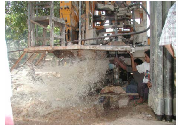
Tubewell developing at Twinma tubewell
