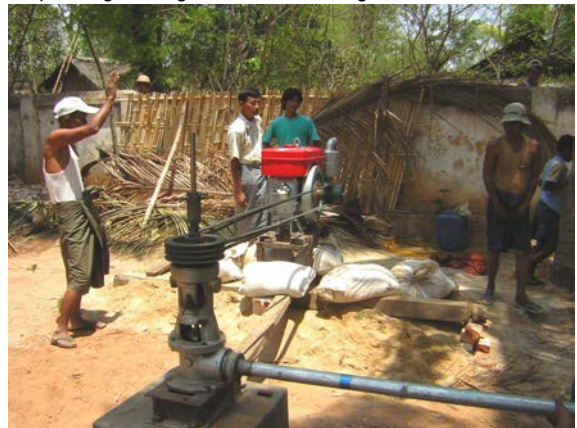
Operating the engine and test running at Twinma tubewell
