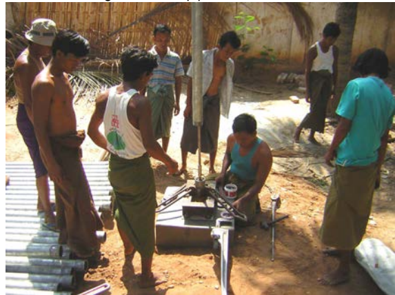
Installing mono riser pipe at Twinma tubewell
