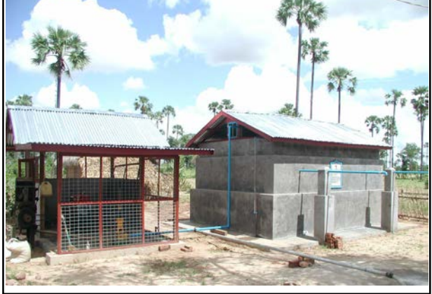
Water supply facilities constructed at Htantawgyi village
