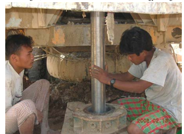
Installing 4"Ø steel screen into the borehole of Htantawgyi village
