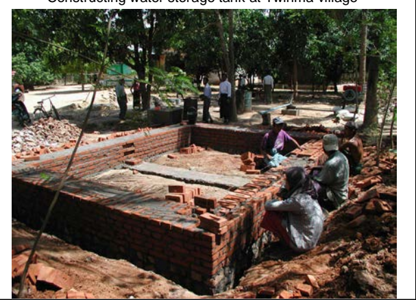
Constructing water storage tank at Twinma village
