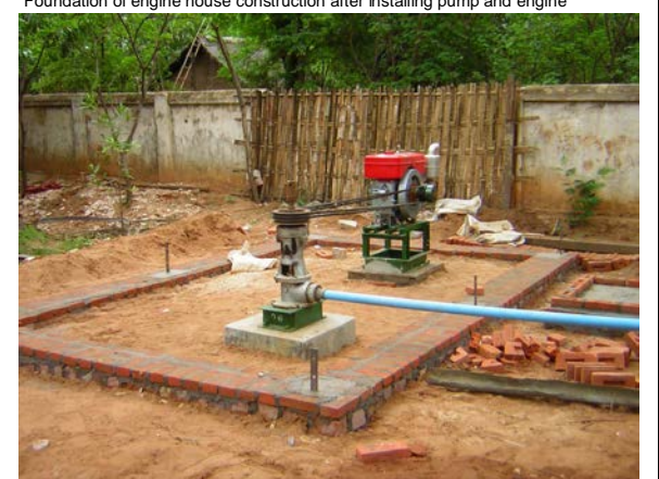
Foundation of engine house construction after installing pump and engine
