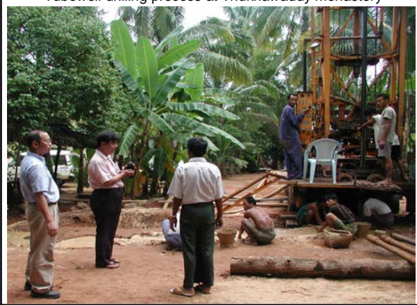
Tubewell drilling process at Thukhawaddy monastery
