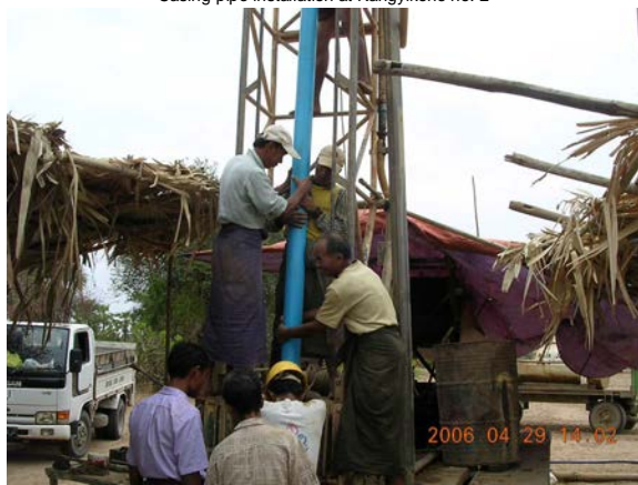
Casing pipe installation at Kangyikone no. 2
