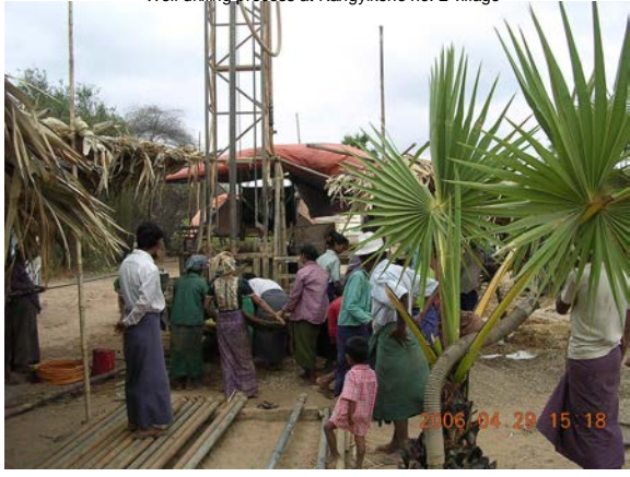
Well drilling process at Kangyikone no. 2 village
