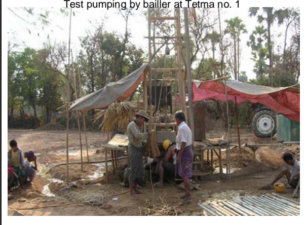
Test pumping by bailer at Tetma no. 1
