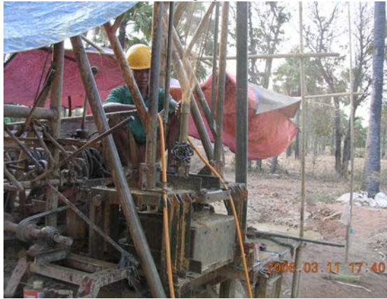
Tubewell developing at Tetma no. 1
