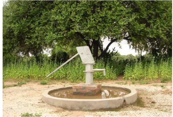
Completion of India mark II hand pump at Kangyikone no. 2 tubewell
