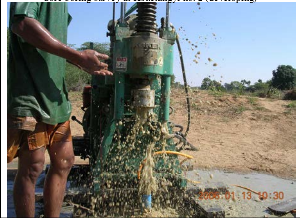
Core boring survey at Konetangyi no. 2 (developing)
