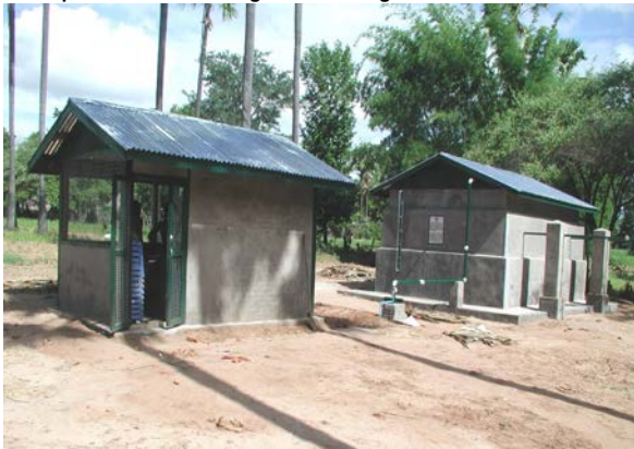
Completion of water storage tank and engine house at Tetma no. 2
