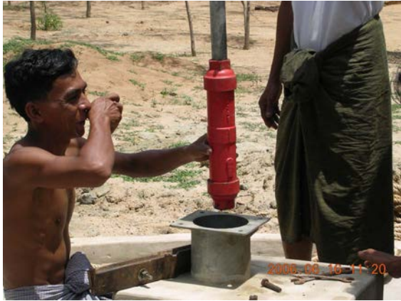
Mark II hand pump installation at Konetangyi village
