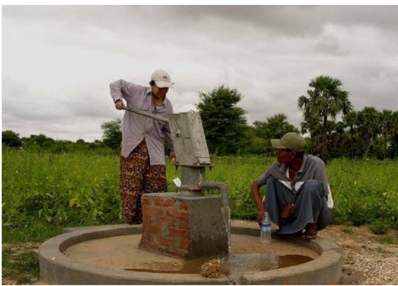
Operating India mark II hand pump at Kangyikone no.3 tubewell
