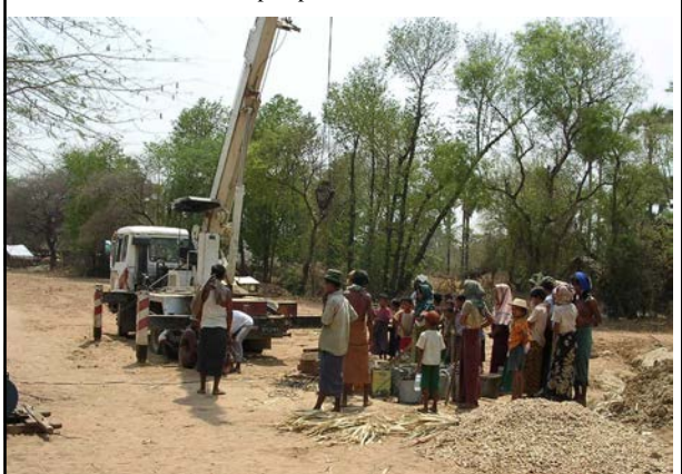
Submersible pump installation at Tetma no. 1
