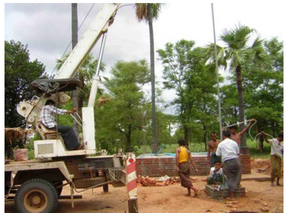
Submersible pump installation at Tetma no. 2
