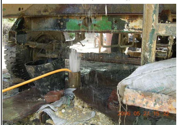
Tubewell developing at Konetangyi no. 3
