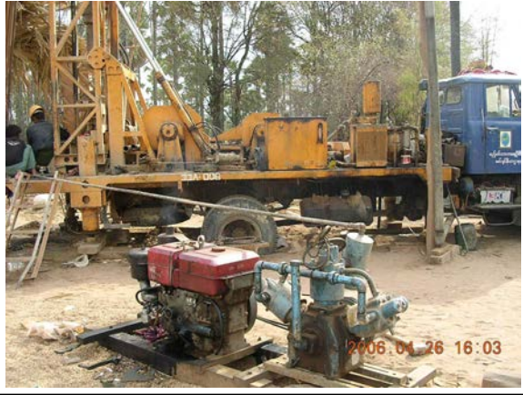
Tubewell drilling process at Tetma no. 2
