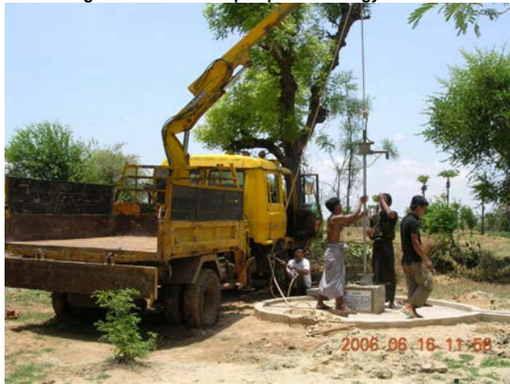
Installing India mark II hand pump at Konetangyi no. 3 tubewell
