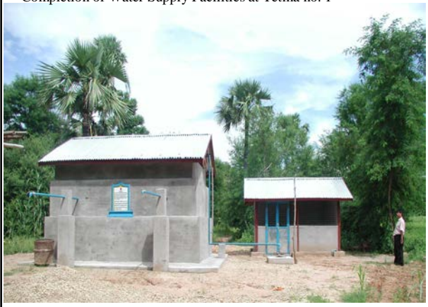
Completion of Water Supply Facilities at Tetma no. 1
