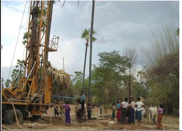
Tubewell drilling by DDA 006 rig at Tetma no. 2
