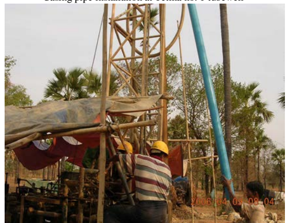
Casing pipe installation at Tetma no. 1 tubewell
