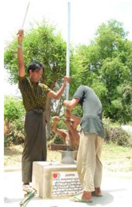
Mark II hand pump installation at Konetangyi village
