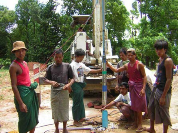
Submersible pump installation at Tetma no. 1
