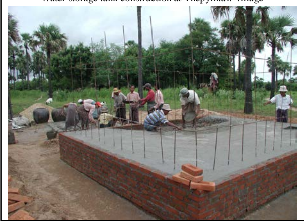
Water storage tank construction at Theypintaw village
